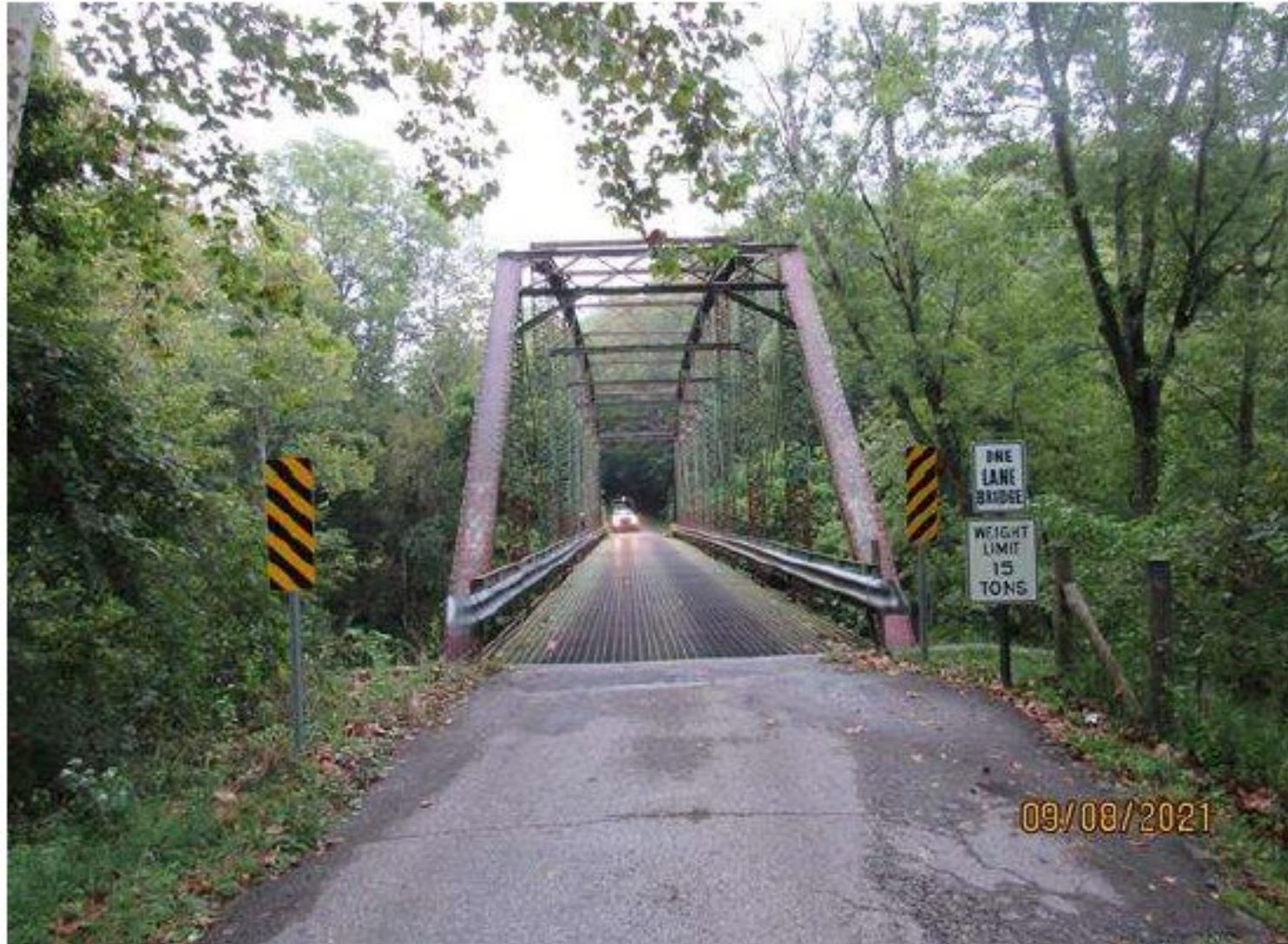
Alignment Looking East (15 Ton, One Lane)
