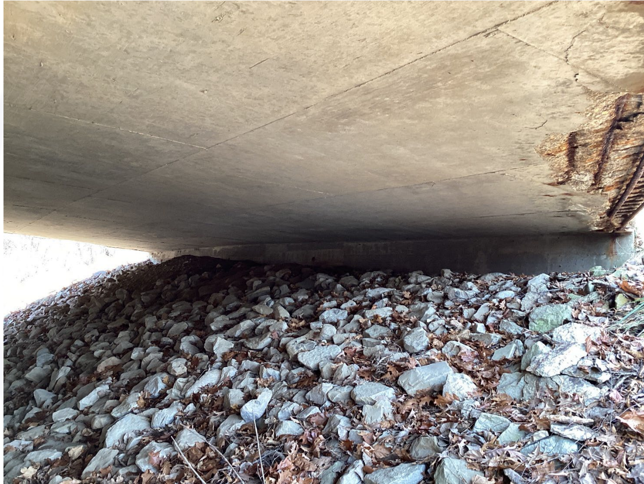
South End Bent and Span A Superstructure
